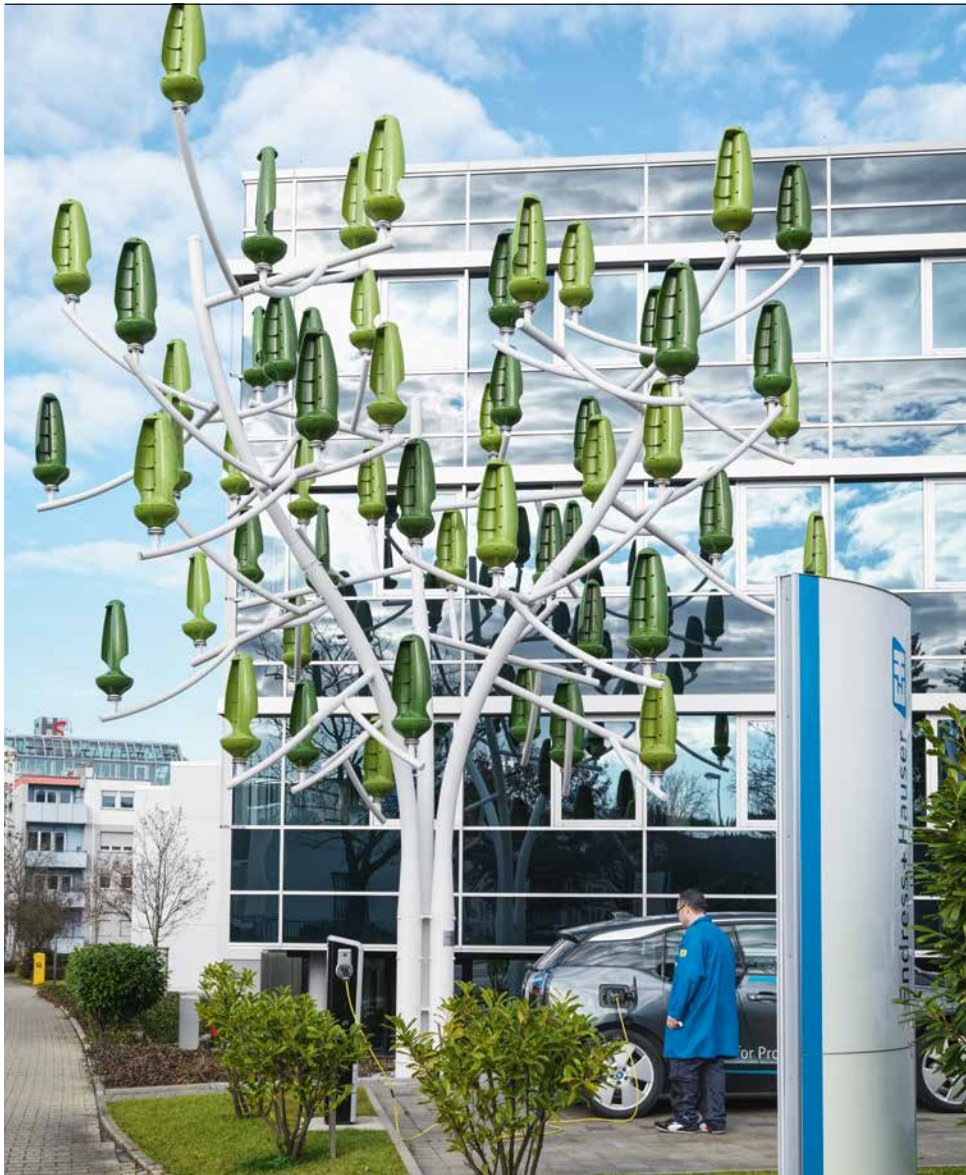
Eco power plant for the city: The wind tree supplies the e-vehicle charging station with electricity.
